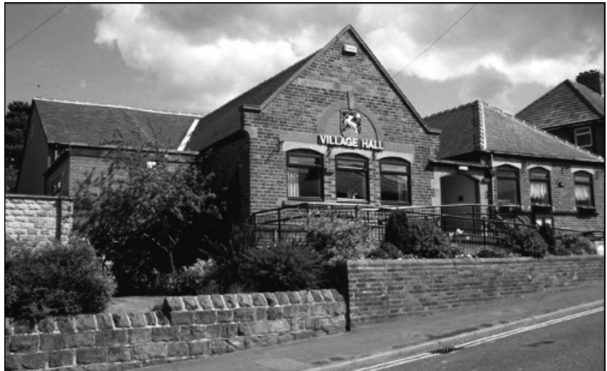
Harthill Village Hall: in need of a bit of TLC
